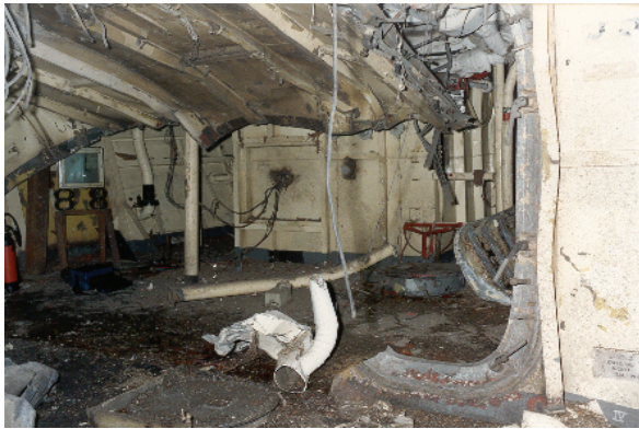
Figure 1 Roofdier Trials internal explosion
